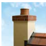
Brick or Stone Chimney (Class 1)
