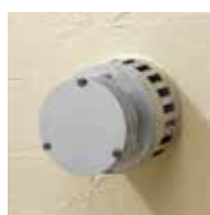
Balanced Flue (No chimney required)
